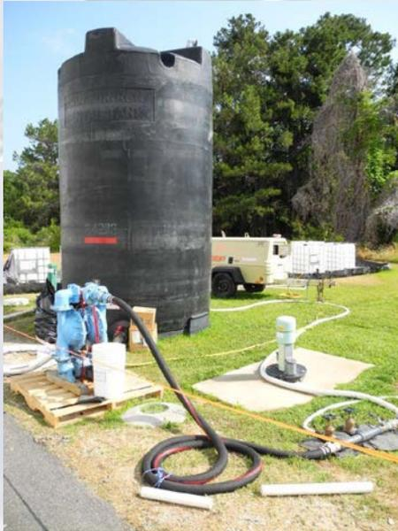
*Injection of the Bioaugmentation Culture into surficial groundwater wells to accelerate biodegradation of VOCs*
