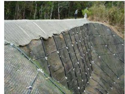
Aerial hydroseeding and Soil nailing projects effectively prevent red soil erosion from impacting Okinawa's coral reef ecosystem. Images here are from a soil erosion control project in the Central Training Area.
