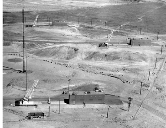
*Athena missile launch complex at Green River Test Site. Climate control shelters are rolled back to expose launcher.*
