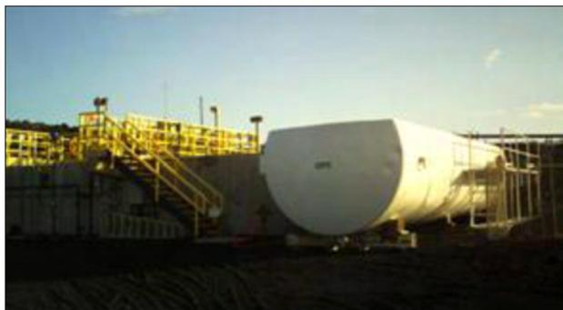
*Old POL Tank Recycled to a Wastewater Plant Pretreatment Basin*
