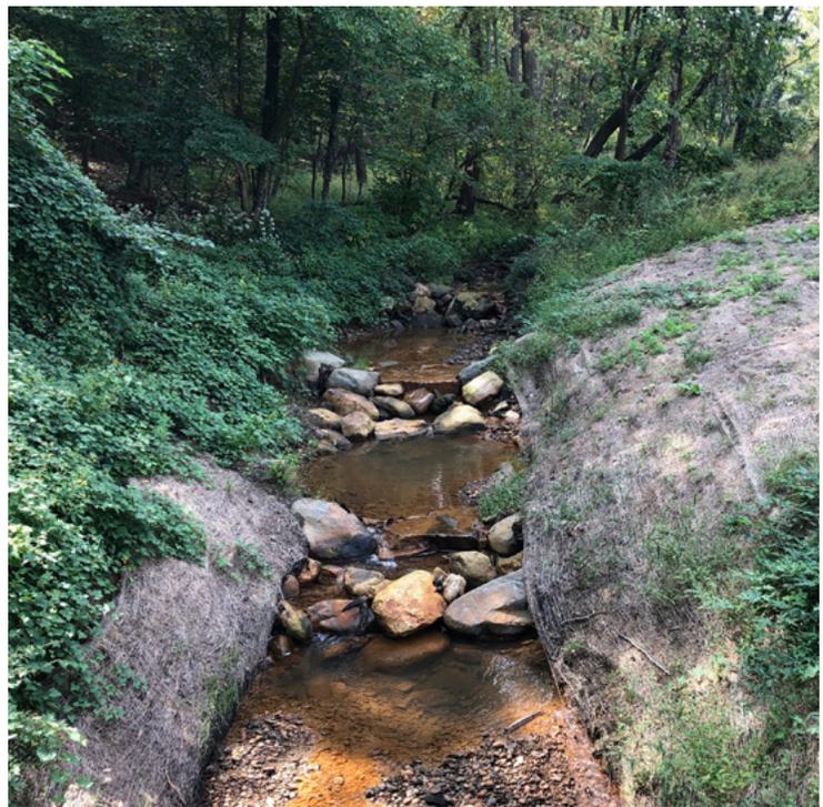
Regenerative step pool constructed as part of a stream restoration at ANC.
