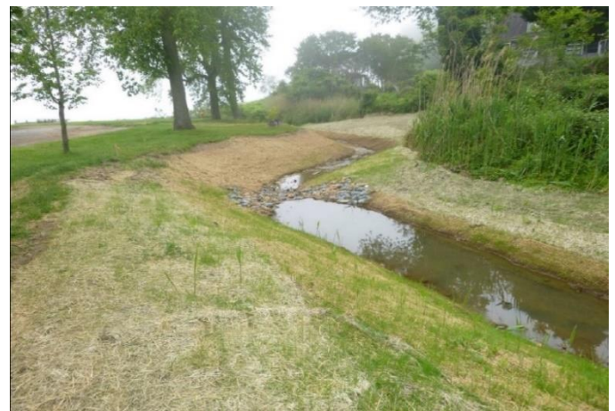
Figure 4. Naval Research Laboratory Chesapeake Bay Attachments conducted stream restoration that repaired stormwater infrastructure, reduced bank erosion and sediment loads, promoted floodplain connectivity and enhanced species habitat.
