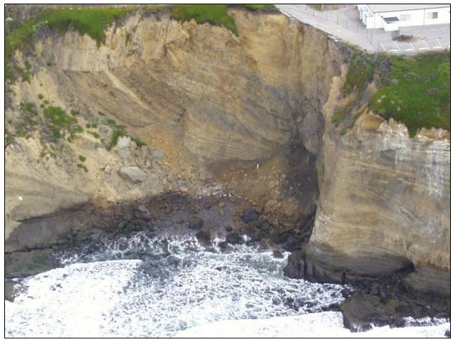
Figure 2-1 Slide area in the western portion of Pillar Point AFS, view to east. This slide threatens Facility 17 at upper right (photographed by J. Carucci, 1998).
