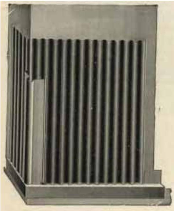
*Illustration 14: An example of corrugated siding, with application beginning at the bottom of the wall (Milwaukee Corrugating Co. 1920:146).*
