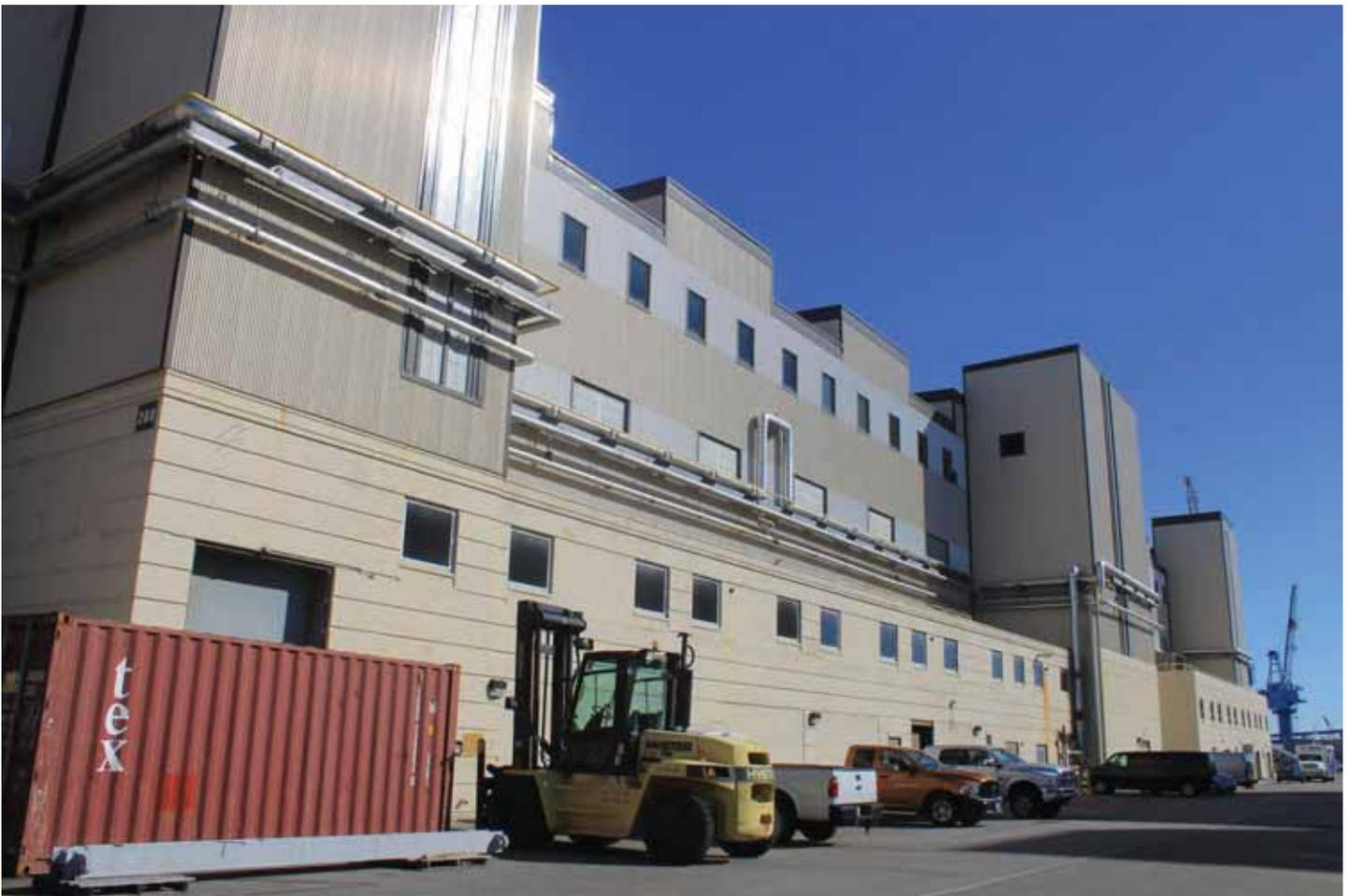
*Illustration 75: Building 268 at NNSY has replacement corrugated metal cladding, which has been painted. As long as the rhythm of corrugation can be retained, in-kind replacement should be considered for any type of corrugated metal (Photographer: Samantha Driscoll 2016).*
