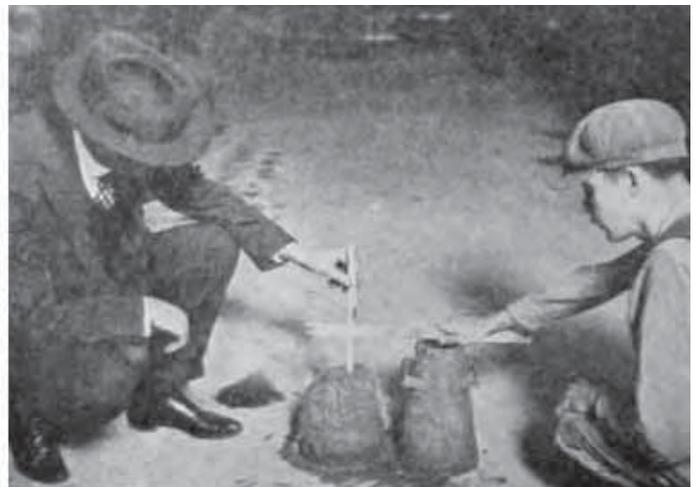
*Illustrations 4 and 5: The images show the “Slump Test” inspection method for cast-in-place concrete, which is conducted on-site (Atlas Portland Cement Company 1927:12).*
