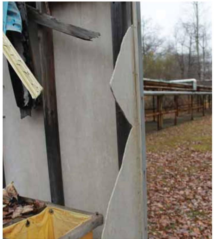
*Illustration 86: Detail of Building 1508 at Picatinny Arsenal where large sections of flat panel asbestos-cement have been broken. Note the thin, brittle nature of asbestos-cement (Photographer: Samantha Driscoll 2015).*
