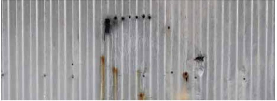
*Illustration 74: Detail of the in-kind material patch on Building 1506. Note the alignments of the corrugations make the patch almost undetectable, but the corroded steel fasteners have caused staining (Photographer: Samantha Driscoll 2015).*
