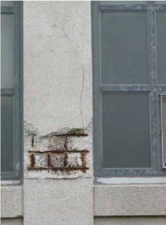
*Illustration 50: The grid of the steel reinforcement is visible on NSFC Building 1, as the rusted steel has caused the delamination and spalling of the surface concrete (Graves 2012).*
