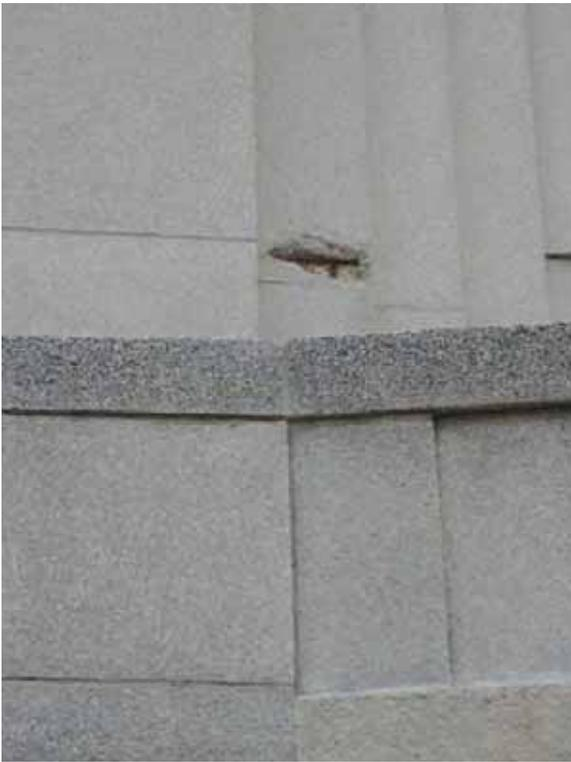
*Illustration 49: A section of rusted steel reinforcement on NSFC Building 1 has resulted in the spalling of the concrete (Graves 2012).*
