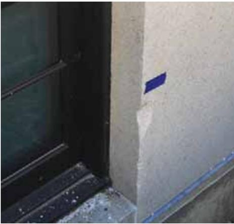
*Illustration 53: An example of spalling on Building 3 at NSA Bethesda. The concrete is undergoing repairs, and the blue tape is used to mark the location of a needed repair (Photographer: Samantha Driscoll 2015).*
