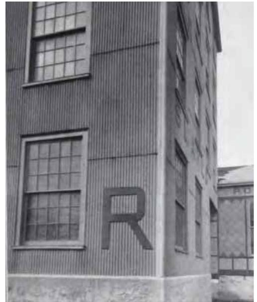
Illustration 36: An example of corrugated asbestos-cement panels as siding on an industrial plant (Asbestos Manufacturing Company 1909:17).
