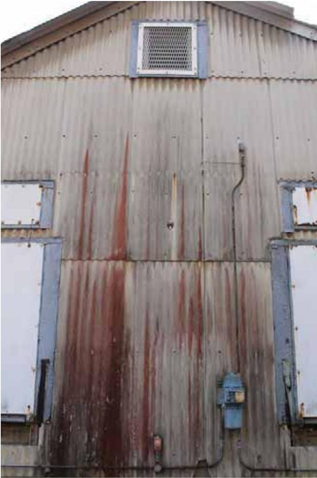
*Illustration 83: The corrugated asbestos-cement cladding has severe stains, indicating lichen growth (Photographer: Samantha Driscoll 2015).*
