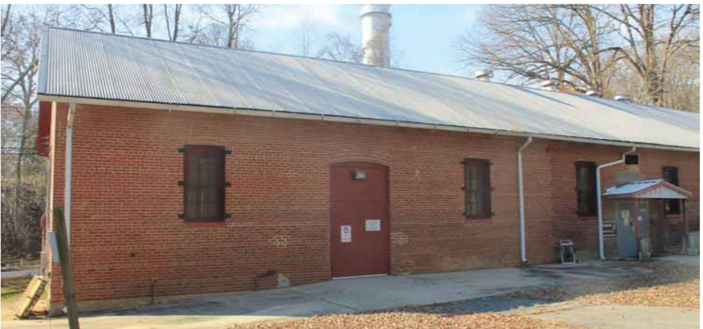
*Illustration 89: Building 160 at NSF Indian Head is an example of a suitable substitute replacement roof. The corrugated asbestos-cement roof was replaced with a corrugated metal roof in 2010 (Photographer: Samantha Driscoll 2015).*
