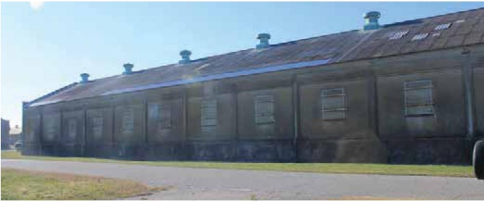
*Illustration 88: Building 74 at NNSY, St. Juliens Creek Annex has several corrugated metal patches on the corrugated asbestos-cement roof. While the replacement patches have similar corrugation widths, the difference in materials is obvious. If the corrugated metal was painted, the patches would blend more with the historic fabric (Photographer: Samantha Driscoll 2016).*
