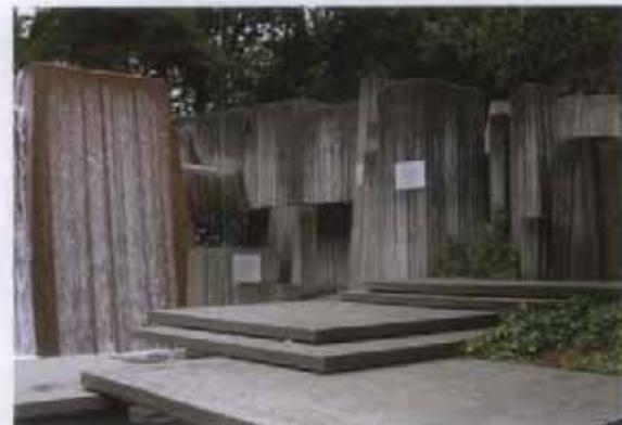
*Figure 9. The Ira C. Keller Fountain in Portland, Oregon, was designed by Lawrence Halprin and constructed in 1969. The fountain is constructed primarily of concrete pillars with formboard textures and surrounding elements, patterned with geometric lines, which facilitate the path of water. Photo: Anita Washko, Wiss, Janney, Elstner Associates, Inc.*
