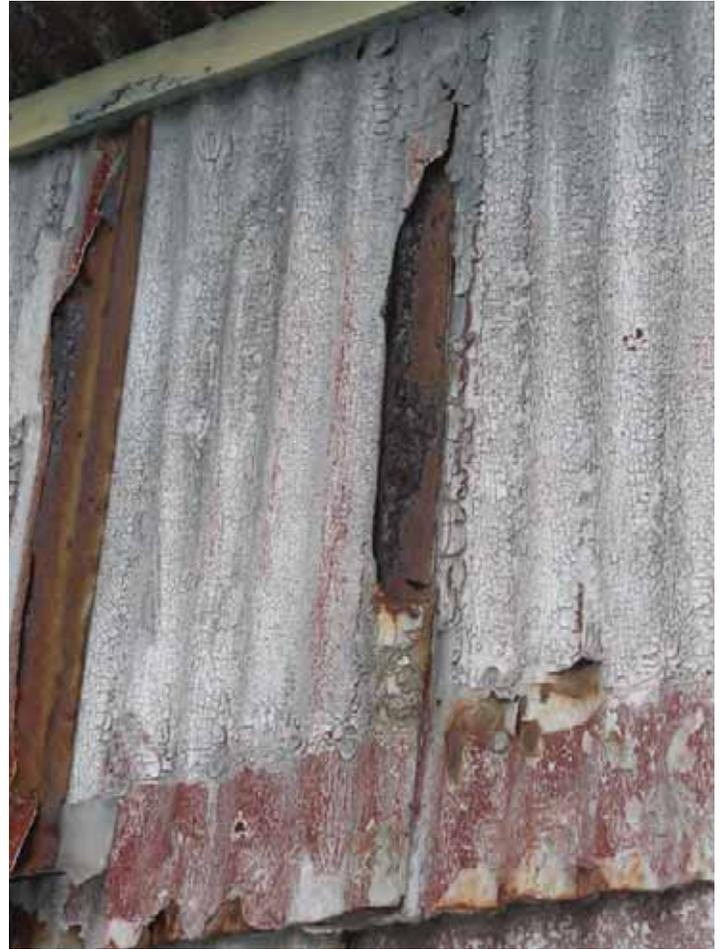
*Illustration 69: Detail of corrosion on Building 1504A. Painting is the primary maintenance of corrugated steel, as it protects the steel from moisture (Photographer: Samantha Driscoll 2015).*
