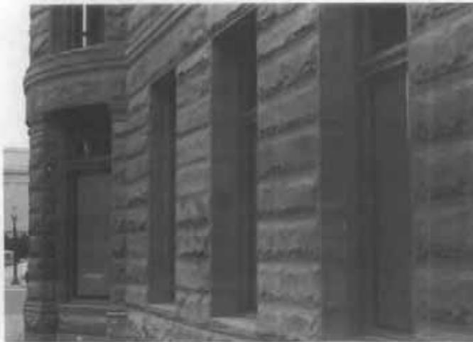
*Illus. 16. The good quality substitute materials shown here do match the historic sandstone in color, texture, tooling and surface details. Dry-tamp cast stone was used to match the red sandstone that was no longer available. The reconstructed first floor incorporated both historic and substitute materials. Sufficient molds were made to avoid the problem of detecting the substitutes by their uniformity. Photo: Sharon C. Park, AIA.*
