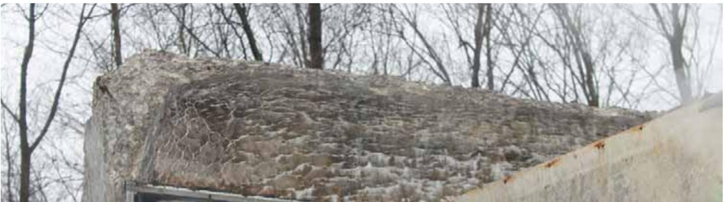
*Illustration 56: Building 1507 at Picatinny Arsenal has a rather extreme example of efflorescence, cracking, and spalling due to moisture infiltration (Photographer: Samantha Driscoll 2015).*
