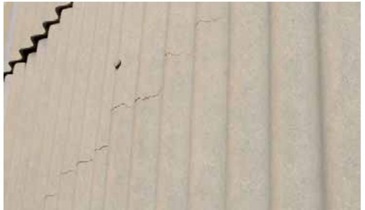
*Illustration 81: Detail of the hairline cracks visible in the corrugated asbestos-cement on Building 448 (Photographer: Samantha Driscoll 2015).*
