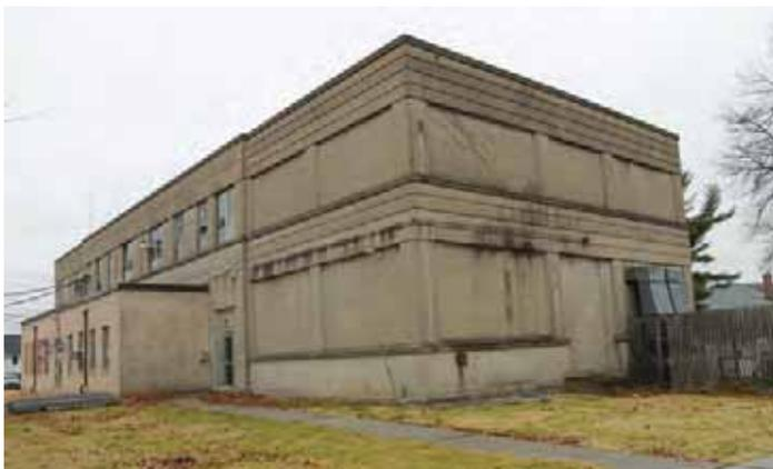
*Illustration 57: Building 173 at Picatinny Arsenal showing staining along concrete. The staining will be removed with a low pressure powerwash with mild detergent, a technique approved by the NJHPO (Photographer: Samantha Driscoll 2015).*
