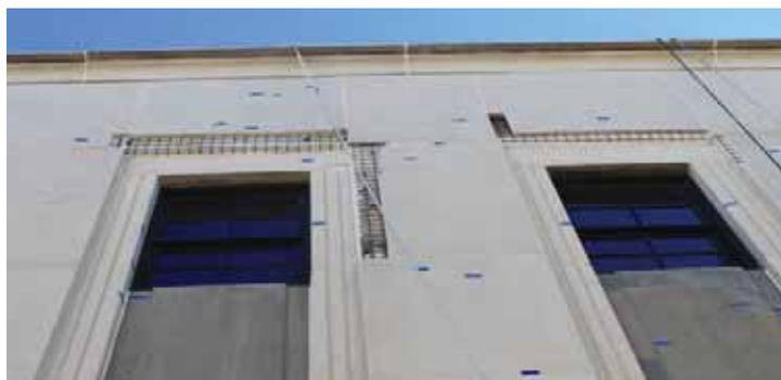
*Illustration 64: Detail of the corroded and exposed steel reinforcement on Building 3, which caused the de-lamination and spalling of the surface concrete. Wire mesh and stainless steel bars will be inserted in these areas prior to patching for stability (Photographer: Samantha Driscoll 2015).*
