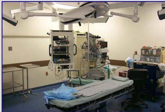
Ceiling-mounted boom racks and flat-panel video displays located on suspended, swiveling racks reduce clutter in OR and allows surgical team to work in neutral postures.
