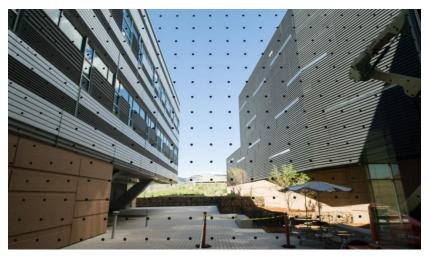
Dot pattern applied to the exterior of a National Renewable Energy Laboratory (NREL) building to help prevent bird collisions. Dots are approximately 1/2" in diameter spaced 2" vertically and horizontally. Photo by Dennis Schroeder, NREL 31193
