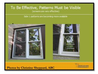
Applying a product to the outer surface (surface #1) of the glass is always most effective. Applying a product to surface #2 or #3 (inner surfaces) can be effective if surface #1 is not so reflective that the pattern beneath is not visible to birds(see Fig. 1).
