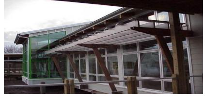
Window netting installed feet from window on slanted wooden beams. Photo by USFWS
