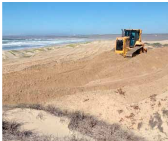
(left): Re-contoured dunes at Surf Beach on Vandenberg Air Force Base, following restoration work in 2014. USFWS (right): Re-contouring of dunes at Surf Beach on Vandenberg Air Force Base in 2014. Photo courtesy of MSRS
