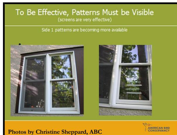
Applying a product to the outer surface (surface #1) of the glass is always most effective. Applying a product to surface #2 or #3 (inner surfaces) can be effective if surface #1 is not so reflective that the pattern beneath is not visible to birds(see Fig. 1).
