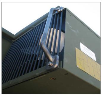
Grabbing the safety handle instead of the angle bracket puts less stress on the wrist tendons when climbing onto the cooling fan housing.
