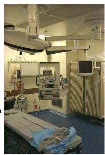
Swiveling racks and height adjustable system eliminate working in non-neutral postures.
