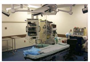
System of ceiling-mounted boom racks and flat-panel video displays located on suspended, swiveling racks reduces clutter in OR and allows surgical team to work in neutral postures.
