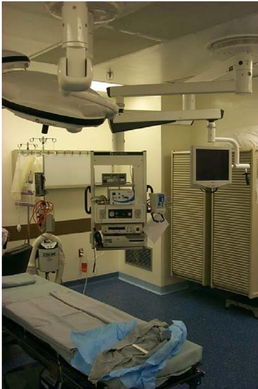
Hospital operating suite renovation with ergonomically designed “Skytron” ceiling-mounted racks raise surgical equipment up off the floor to eliminate operating room clutter and improve work flow. In addition, flat panel video endoscopy TV monitors and a local exhaust surgical smoke extractor were installed on these boom arms.
