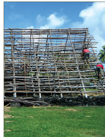
Hale repaired using in-kind materials
