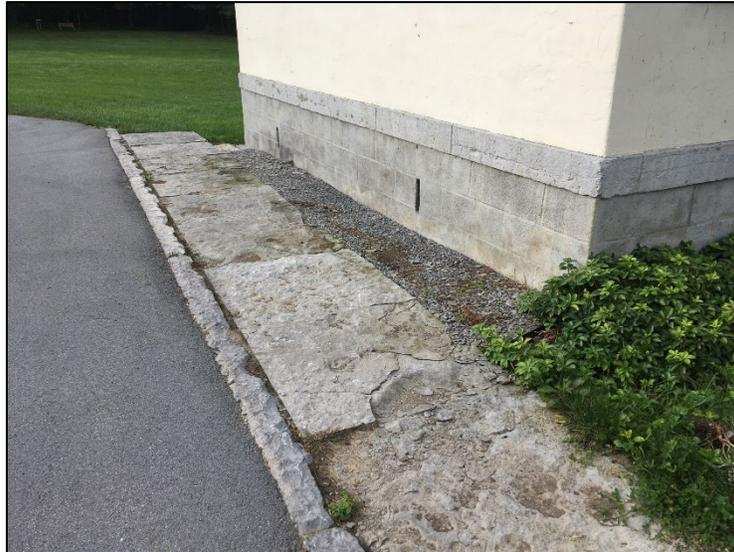
Figure 53. Photograph showing the deteriorating Trenton Limestone pavers (Fort Drum). This material does match our local limestone, but in this form, it is too friable to serve as a walkway. Some of the pavers cracked during installation, others began to deteriorate during the first freeze thaw cycle after installation. Deterioration was exacerbated dramatically by use of de-icing material, but the walkway was too dangerous to be cleared by using only manual snow and ice removal methods.
