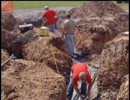
The NDCEE geothermal technology demonstration at Fort Indiantown Gap will help PANG achieve energy-independent facilities, one of its five strategic objectives for facility sustainability. This photo shows workers installing horizontal and vertical pipes for the heat pump system.
