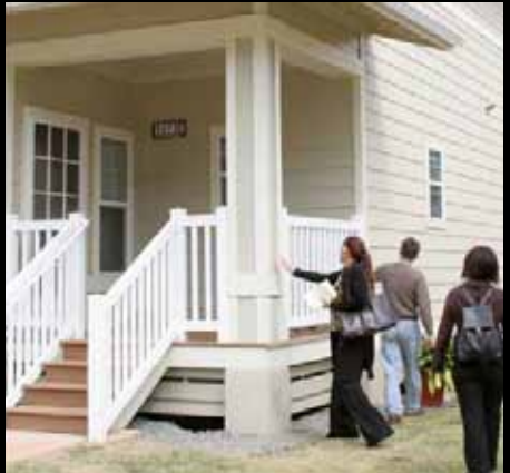
Attendees of the Sustainable Installations Information Exchange were invited to see (and feel) a unique house coat demonstrated on military housing. For the demonstration, a ceramic paint additive was added to house paint to create a coating that radiates solar and ultraviolet rays back into the atmosphere.
