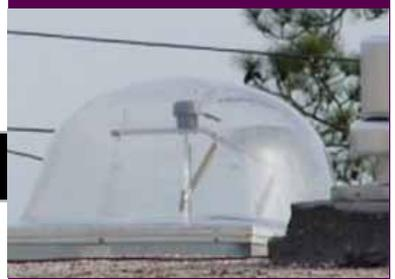
The dome, mirror, and tracking mechanism of a SunTracker ONE system is mounted on the roof of the DPW building at Fort Bragg, NC. A solar cell powers the tracking mechanism that controls the mirrors to optimize the sunlight transmitted to the lobby below.
