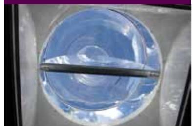
The picture above shows the SolaTube installed in Fort Bragg's Customer Service Conference Room before the diffuser was installed. The SolaTube is segmented for easy installation. The baffles here are in the open position.
