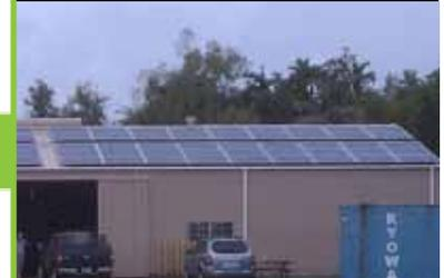
*Before the photovoltaic array was installed at Camp Katuu, PACOM and A/249th Engineering Battalion designed and incorporated modifications to reinforce the roof to support the additional weight of the solar panels and mounting equipment, currently estimated to be 10,500 pounds.*
