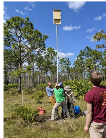
Figure 3. Pour concrete and water into the hole and set with a level.
