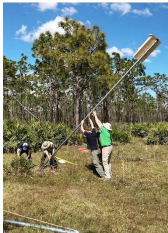
Figure 2. Raise the pole and roost into vertical position.
