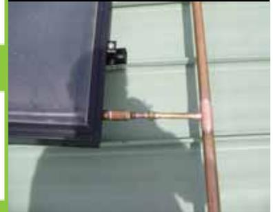
*Solar panels attached to existing metal roof with special clips*
