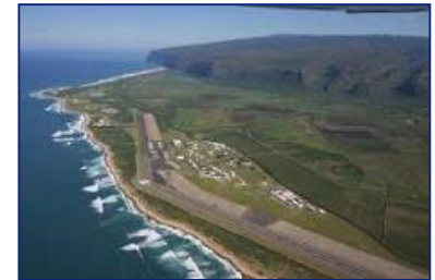
Pacific Missile Range Facility, HI
