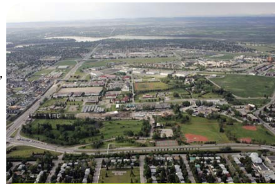
Imbrium Stormceptors play a key role in the sustainability of Currie Barracks
