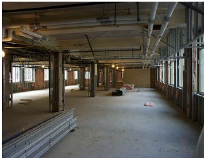
With 7,748 windows and relatively small distances between exterior walls, the Pentagon has a great opportunity for daylight penetration and connection to the outdoors for occupants.
