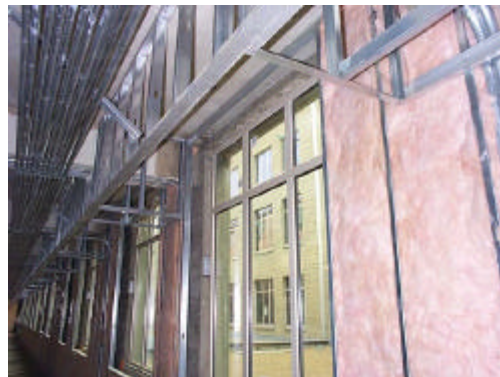
New windows and insulation in Pentagon walls
