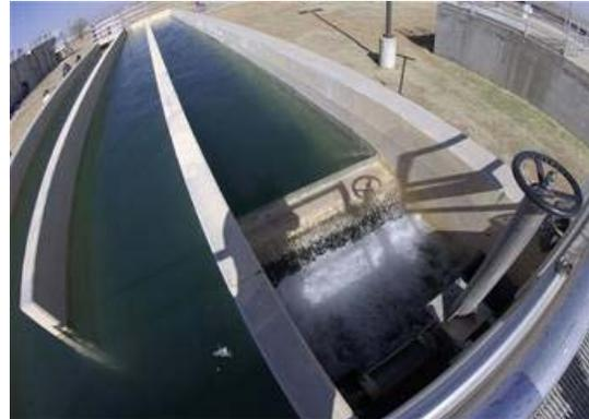
CANNON AIR FORCE BASE, N.M.-- At the 27th Special Operations Wing Waste Water Treatment Plant, water is being chlorinated and then released into the Playa Lake, Apr. 22. Before the water is discharged into the Playa Lake, it undergoes a chlorination process in the chlorine contact chamber. The chamber ejects water approximately every three hours, adding up to a total of 10 discharges per day. (U.S. Air Force photo/Airman Maynelinne De La Cruz)
